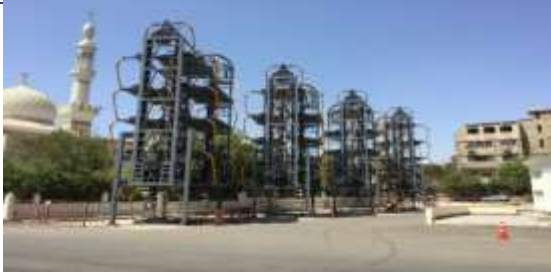
Figure (9a) Illustrating an example for using automated parking structure neglecting any contextual and aesthetical aspects [1].
