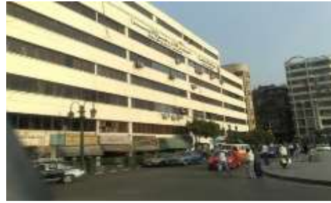
Figure (9b): Old form of parking structures; dull and ugly buildings constitute a source of visual pollution in cities. Opera Garage in downtown Cairo [1].
