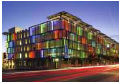
Figure 10 b : Santa Monica Civic Center parking garage, USA
